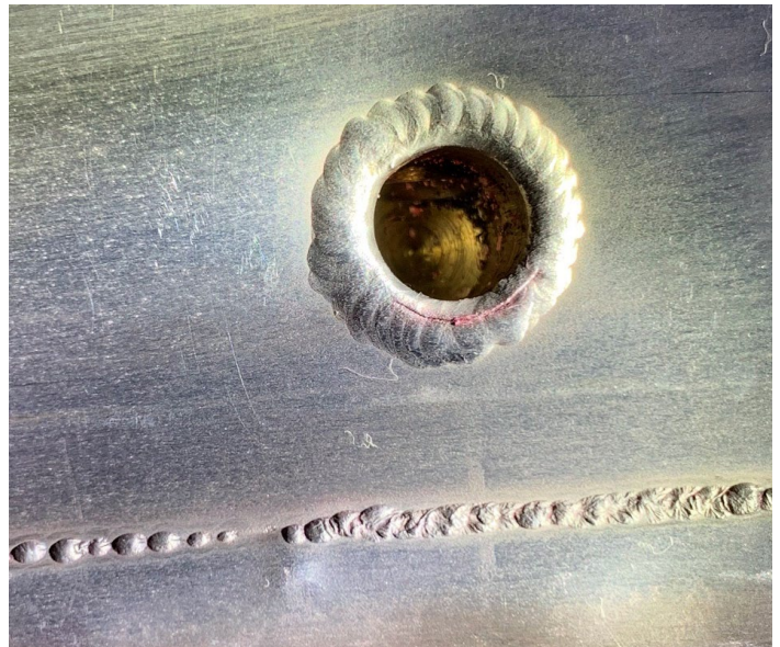
21 22 23 24 25 26 27 28 Red dye indicates a crack in the weld
